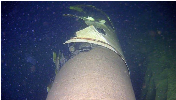
Figure 3. The damaged offshore Balticconnector gas pipeline (Estonian Public Broadcasting, 2024).
